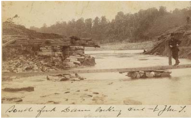
A heretofore unknown photo from the Beale collection, showing the remains of the South Fork Dam after it failed, causing the 1889 Johnstown Flood.
